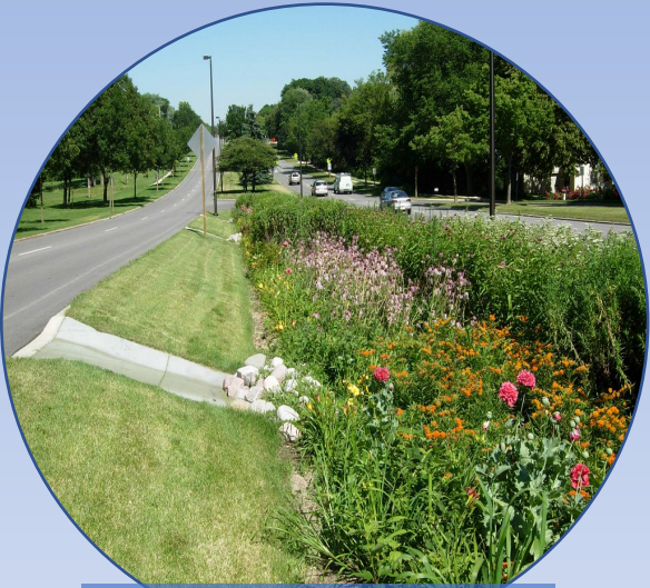
BIORETENTION SWALE
