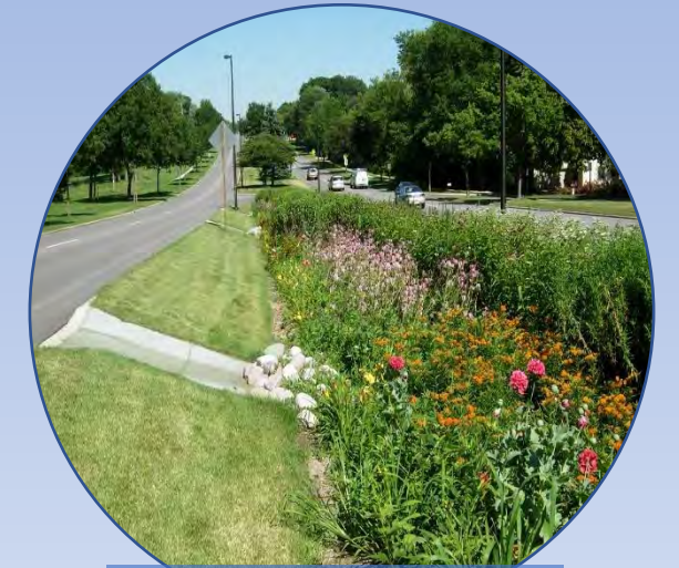
BIORETENTION SWALE
